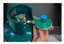
Screw the gas regulator into the valve of the cylinder and, by hand, turn the bolt. Help yourself with a special key for gas regulator for perfect tightening and for avoid damaging the valve gasket compromising the watertight seal.
